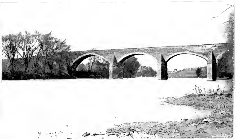
MONOCACY STONE BRIDGE BALTIMORE PIKE
